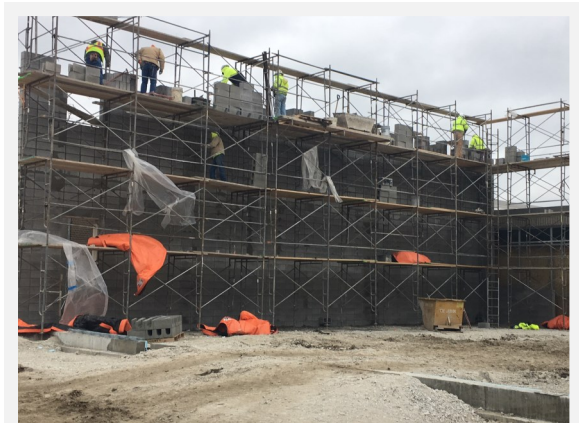
ES - Erection of CMU Bearing Walls
