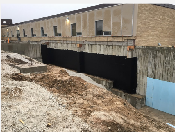
MHS - Completed "Tall Walls"
